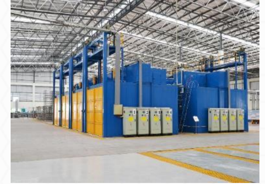
Plate solidification and drying
